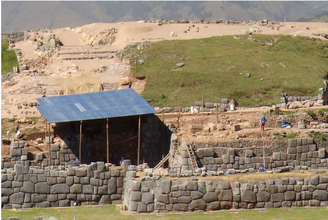
Figure 1: Collapsed portion guarded by roof with impermeable clay layer (above-left) (Miksad, 2012)
