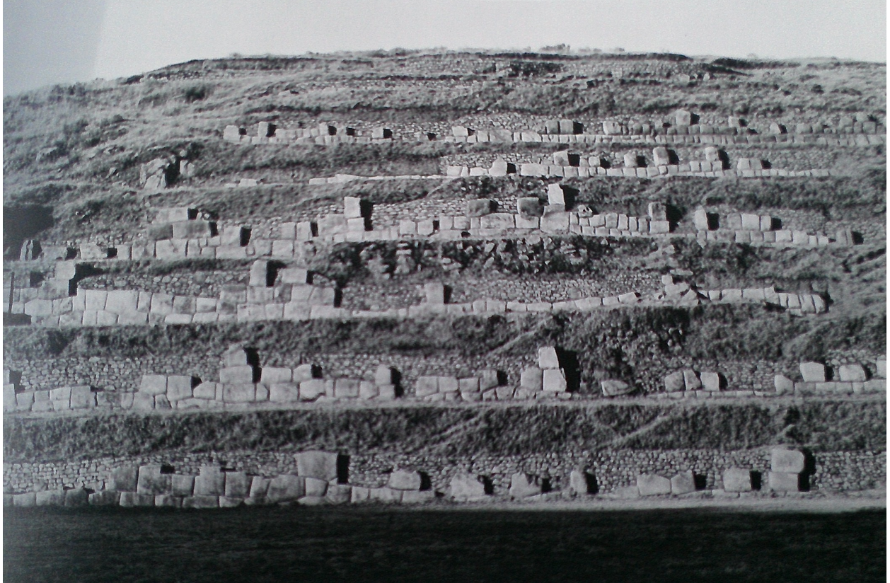
Figure 4: Retaining walls on the south-western side of Rodadero Hill (Hemming, 2010, p. 75)
